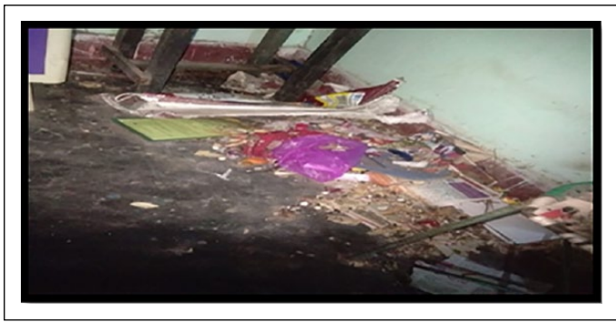
Figure 3. Damage caused by rats.
